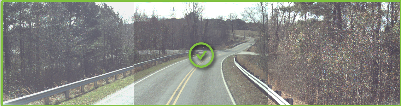
A prototype system for assessing road safety successfully detected guardrails 90% of the time (shown here) and utility poles 88% of the time. Copyright RENCi at UNC-Chapel Hill
